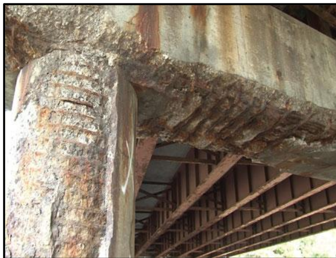
Figure 4: Significant damage from many years of salt and deicing chemical use from a leaking expansion joint. Source: Bridge retrofit using fiber reinforced polymer, cenews.com
