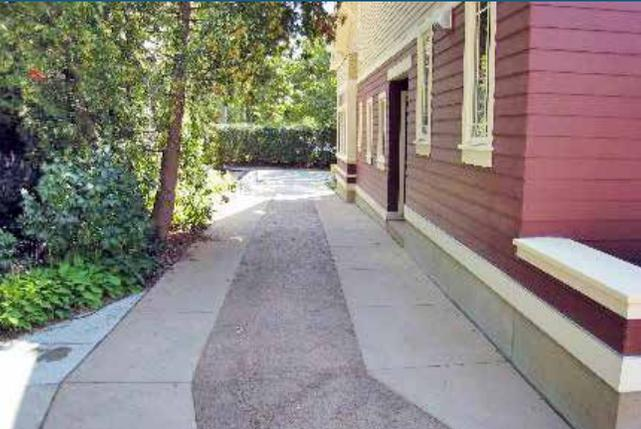
Permeable surfaces include paving systems that allow rainwater to percolate into the ground underneath. They can significantly reduce runoff from parking areas, drive aisles, pedestrian paths and plazas.
