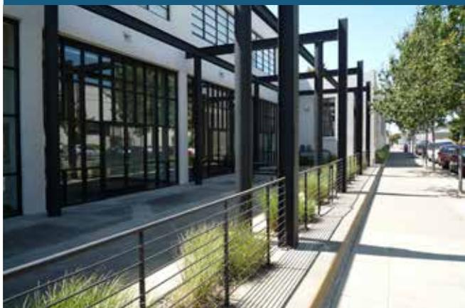
A stormwater planter is a specialized planter system installed adjacent to a sidewalk to manage street and sidewalk runoff. The planter is lined with a permeable fabric, filled with gravel or stone, and topped off with soil, plants, and sometimes trees.
