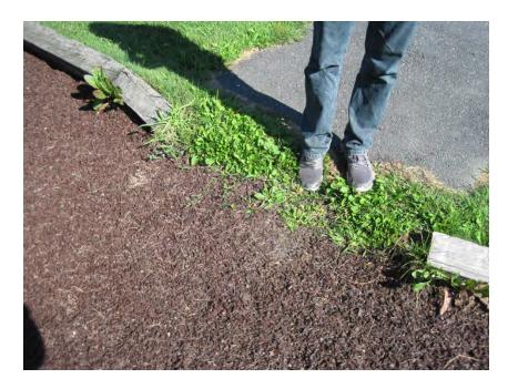
At the bottom of the path, the connection to the playground has a large gap that would make wheelchair transitions difficult.
