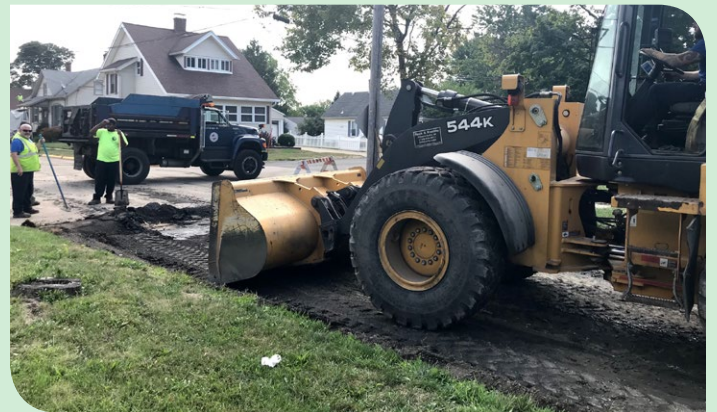
Milling and filling on Follett Street ▲
