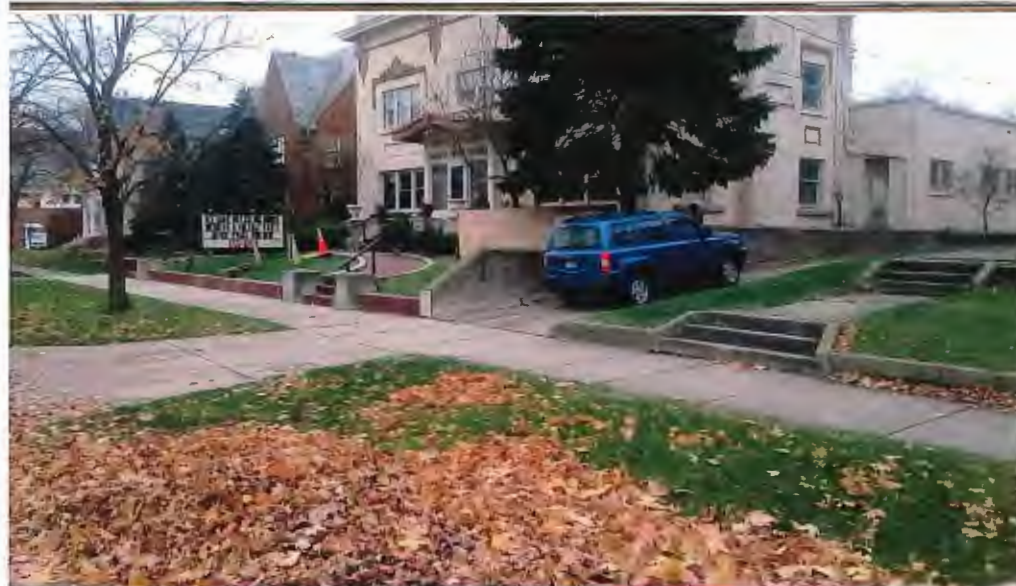
Photo Shows Difference in Grade between Two Properties. Vehicle in Adjacent Drive is Substantially Lower Affecting Sightlines of Pedestrians. Driver's View Is Further Reduced by Existing Tall Concrete Wall..
