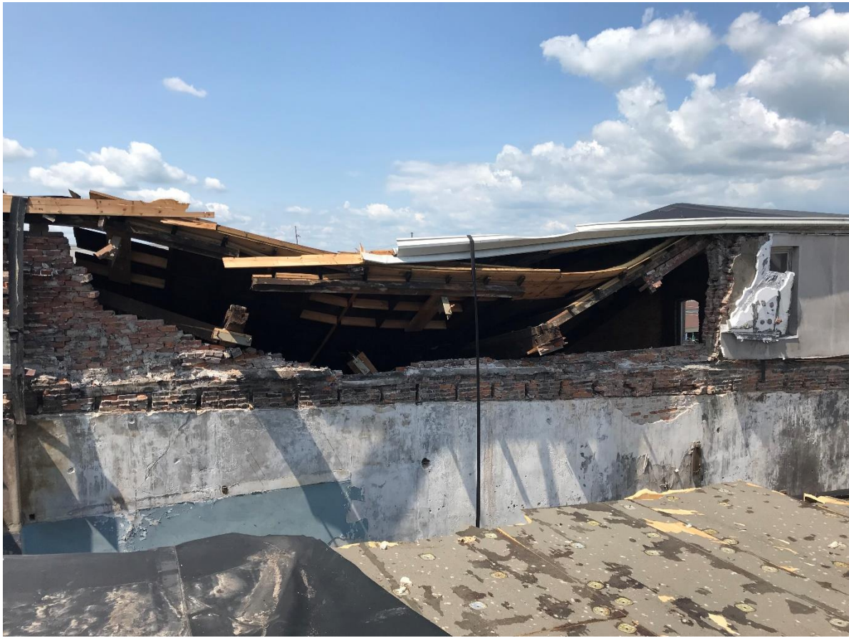
East Wall Storm Damage (before cleanup) (Note roof missing on adjacent building in foreground)
