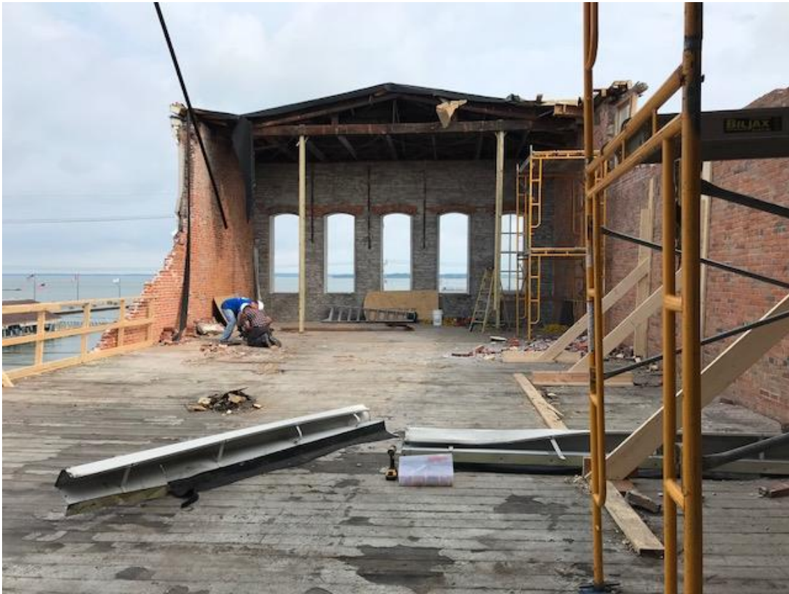
Third floor after damage cleanup Note extent of damage to west wall compared to east wall
