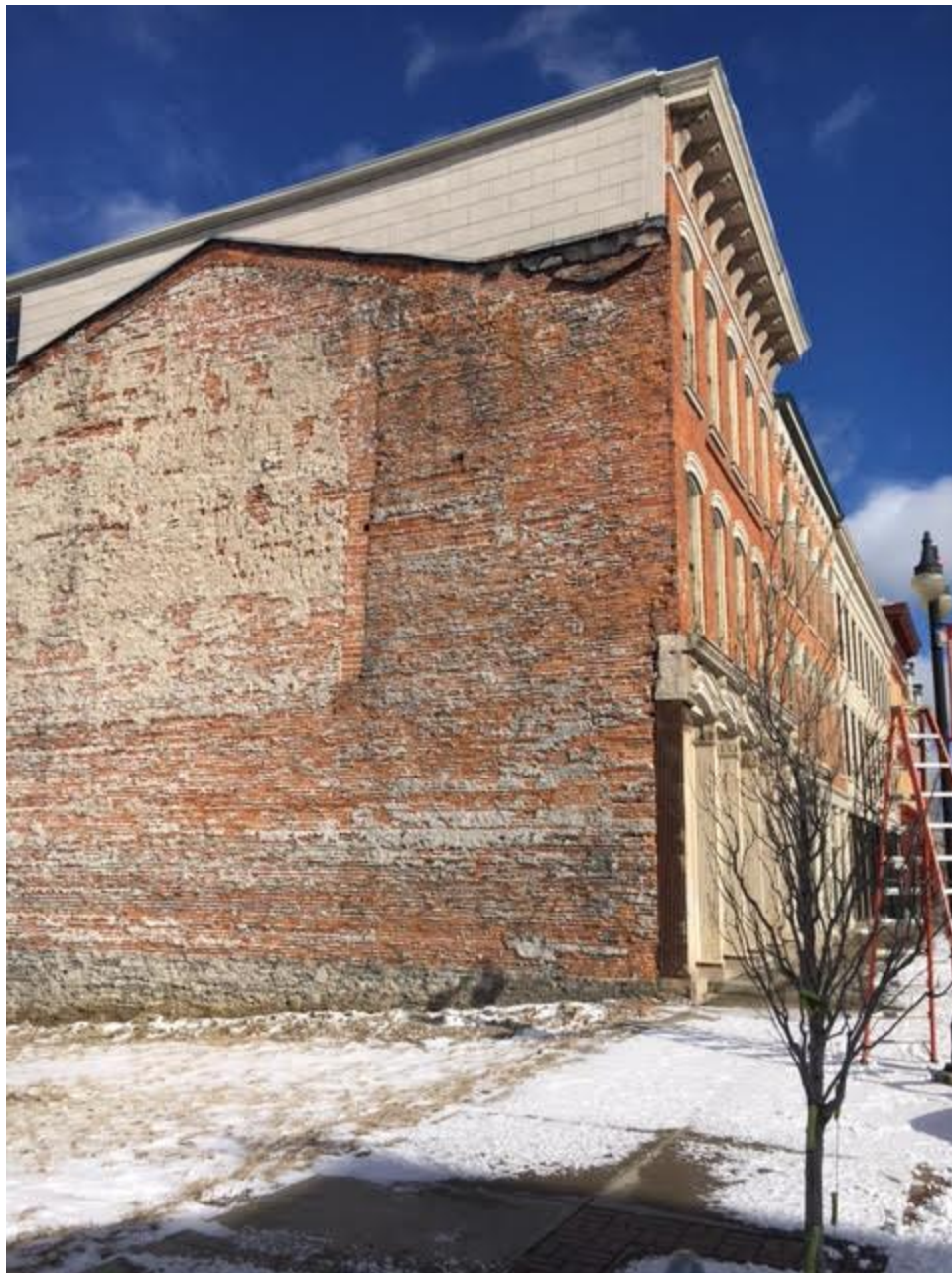
West wall exposed after adjacent building wall demolished Note variation in brick
