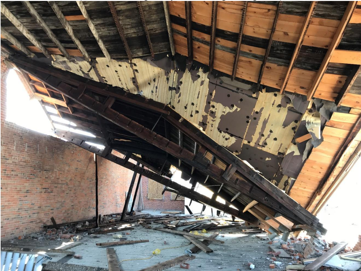
Roof Structure resting on third floor (before cleanup) Note east wall damage with truss ends resting on remaining wall
