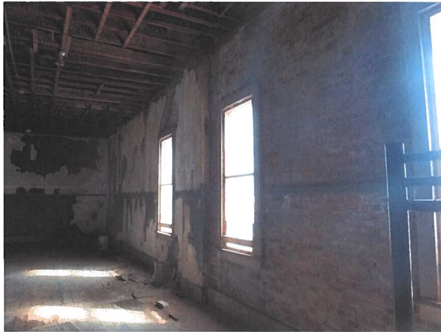
Deteriorating Masonry Wall
