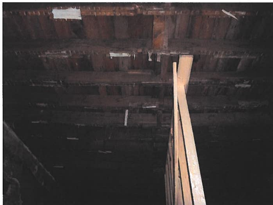
Temporary Floor Joist Support
