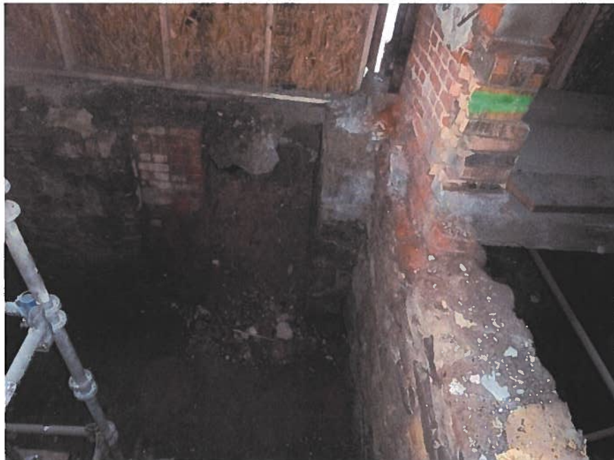
Failing Basement Retaining Wall
