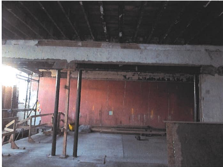
Removed Masonry Bearing Wall Location
