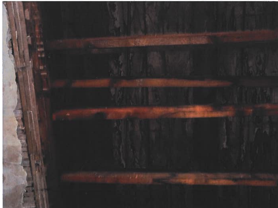
Water Damage to Roof Structure
