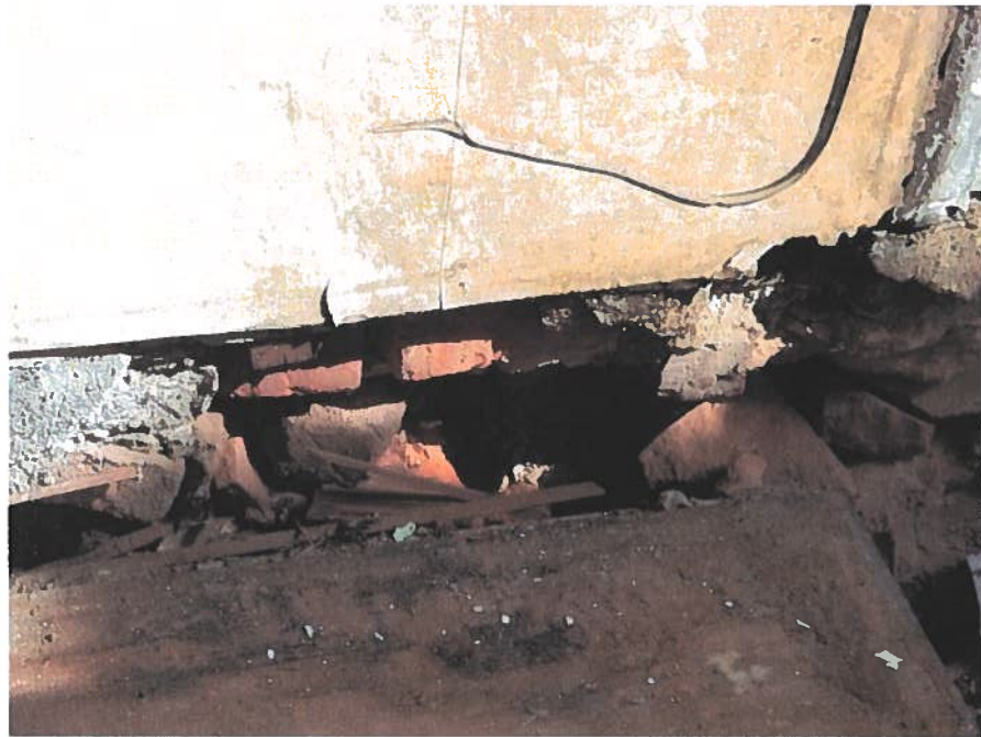
Failing Masonry Walls
