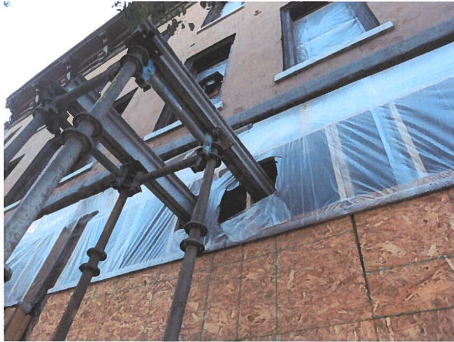
Temporary Wood Beam Support
