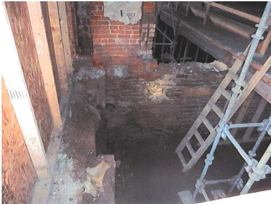
Failing Bearing Wall
