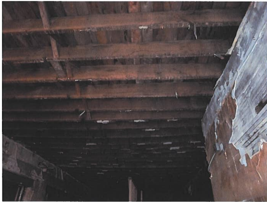
Notched Floor Joists
