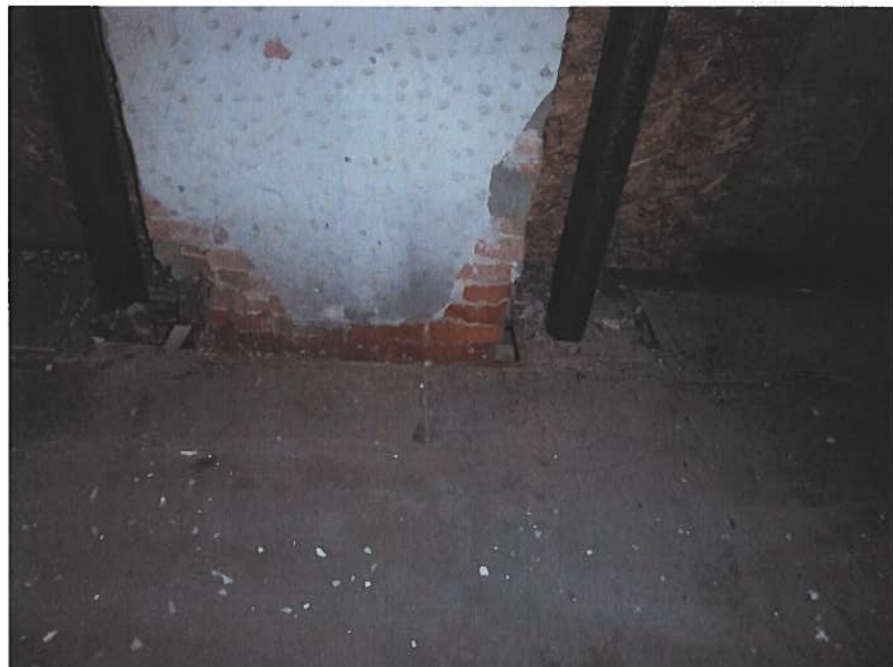
Deteriorating Masonry
