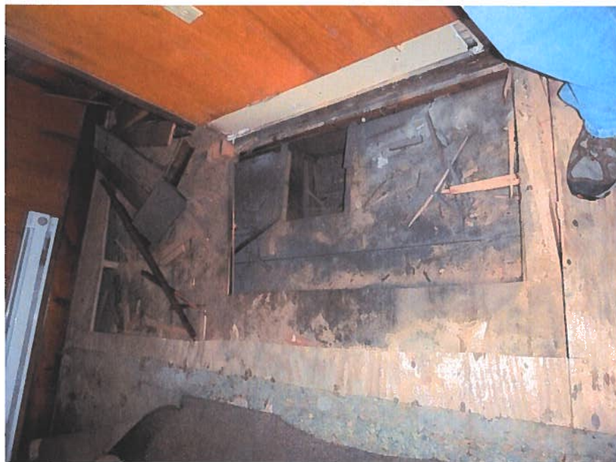
Multiple Floor Layers
