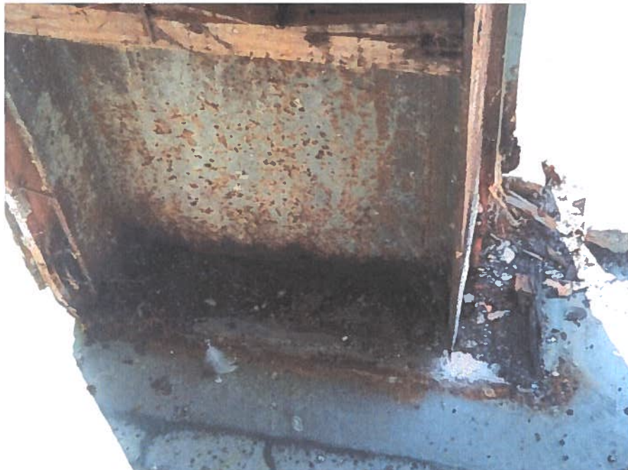
Failed Column Base
