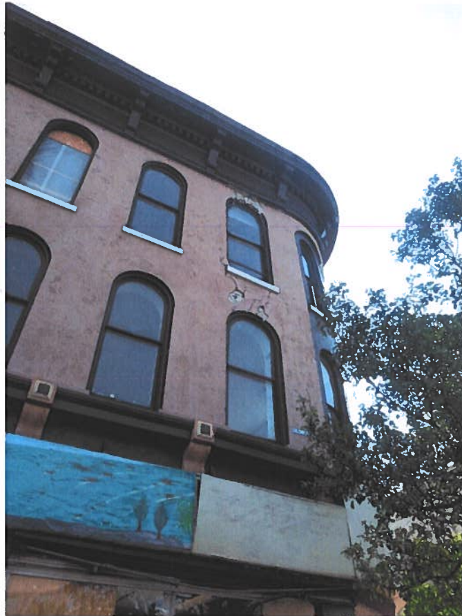
Failing Masonry
