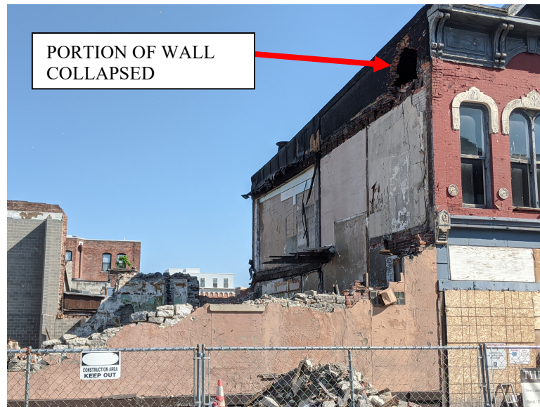
Figure 1 - West bearing wall and south facade wall
