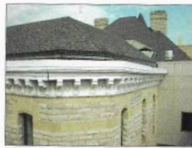
PHOTO OF CORNICE TO BE REPLACED
