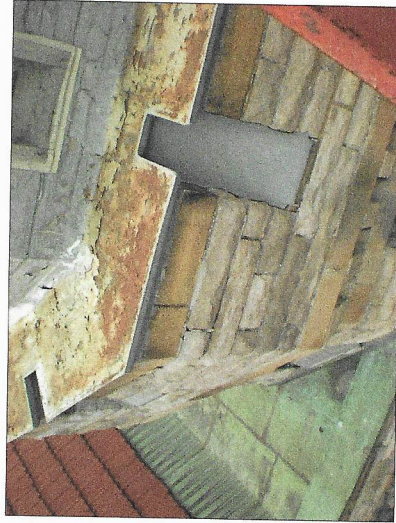
PHOTO OF SHEET METAL TO BE REPLACED WITH BIRD SPIKES
