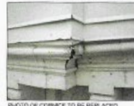
PHOTO OF CORNICE TO BE REPLACED
