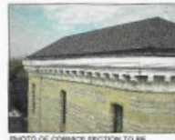
PHOTO OF CORNICE SECTION TO BE REPLACED
