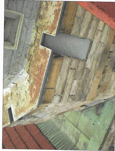
PHOTO OF SHEET METAL TO BE REPLACED WITH BIRD SPIKES
