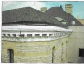
PHOTO OF CORNICE TO BE REPLACED
