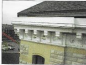
PHOTO OF CORNICE TO BE REPLACED
