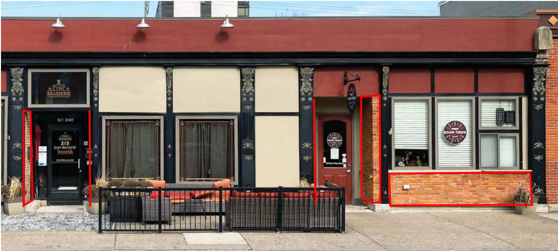
Areas of Exposed Brick to be Painted
