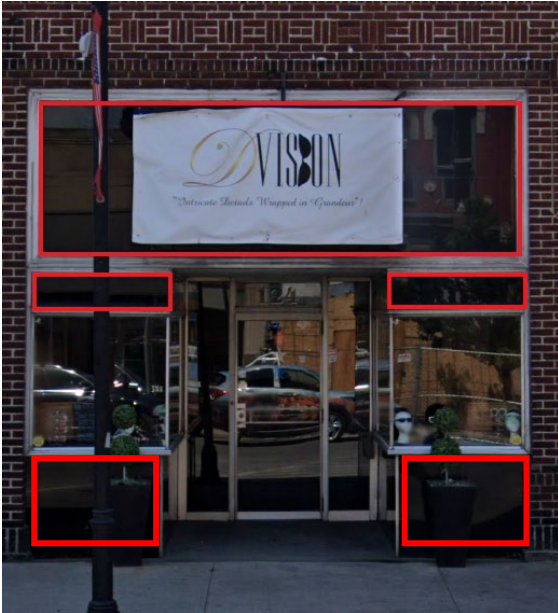
Existing Porcelain Panels
