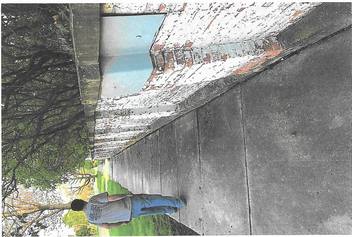
FAILING BRICK WALL TO BE REMOVED
