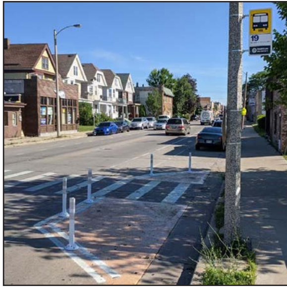
FIGURE 2 Curb Extensions: Curb Extensions are used for pedestrian safety to slow vehicles and shorten the distance to cross the street. (STREETWISE MKE n.d.)
