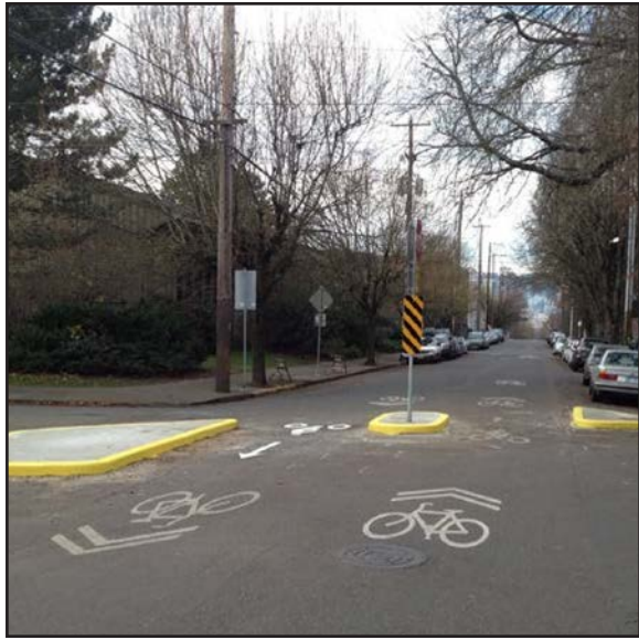
FIGURE 3 Street Diverter: These prevent motor vehicle traffic from continuing straight along the route while still allow people walking and biking access.(STREETWISE MKE n.d.)
