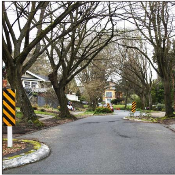
FIGURE 6 Chicane: A series of alternating curb extensions that form an "S" shape to encourage drivers to slow down. (STREETWISE MKE n.d.)
