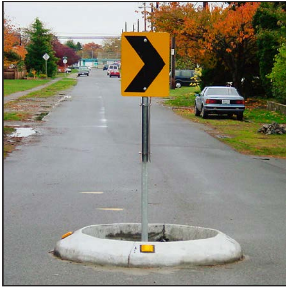
FIGURE 7 Traffic Circle: A structure in the middle of an intersection that forces drivers to slow down and travel in a counterclockwise direction. (STREETWISE MKE n.d.)
