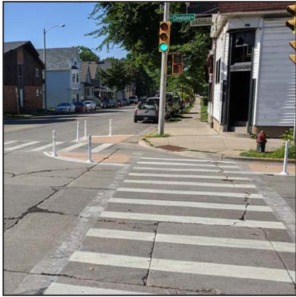
FIGURE 1 High Visibility Crosswalk: A series of pavement markings that define crosswalks and prompt vehicles to yield to pedestrians. (STREETWISE MKE n.d.)
