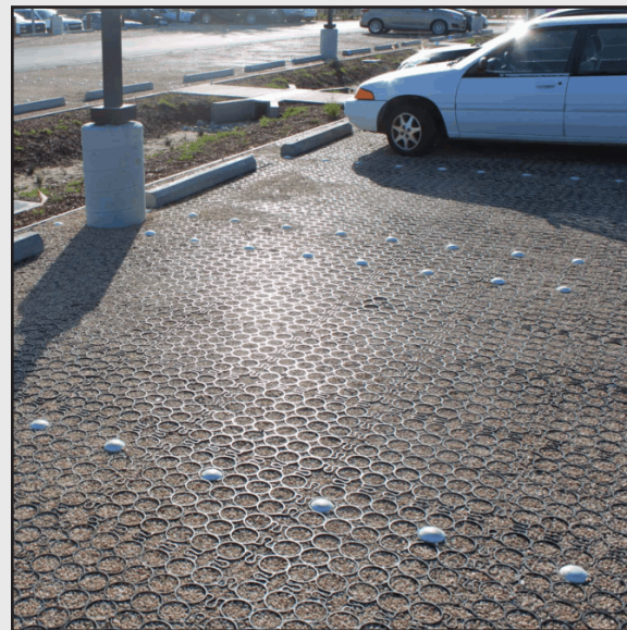
Figure 3: Eco-Paved Parking Lot: This permeable paved parking lot is an example of development something like the Go Green Project can create. (TrueGridPaver, 2017).
