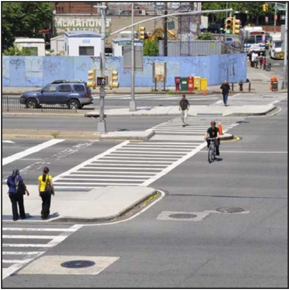
FIGURE 4 Pedestrian Islands: Pedestrian islands are used on wide roadways to allow pedestrians to cross the street one half at the time. (STREETWISE MKE n.d.)
