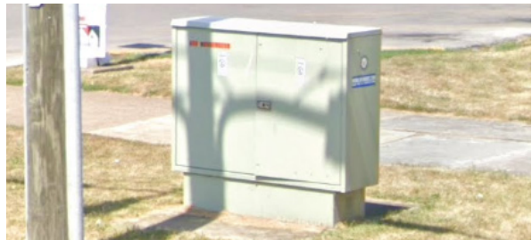
Example of a traffic control utility box.
