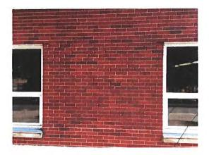
9. Upper Roof windows. Install end dam on the outside of the lentils where the existing flashing ends. Tie in with new sealant.
