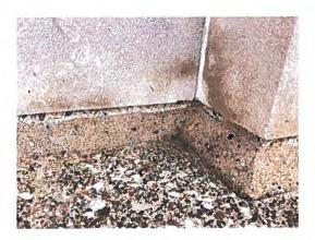
3. All windows inside stone (aluminum to stone) sealant removed and replaced with new.
