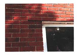
10. Upper Roof Area (3 walls) - old roof line (existing sealant) removed and replaced with mortar.
