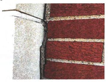
• Remove and reinstall 100% mortar in all limestone top bands surrounding the entire perimeter of the building.
