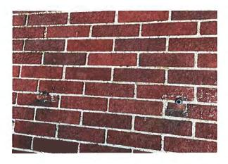
13. Penetrations with deficiencies, holes or damage. Apply new sealant where needed.
