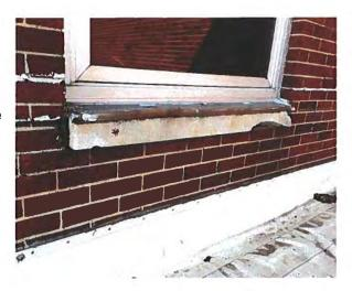
12. Upper Roof Area – North side wall has 4 holes. Do not remove, apply sealant over to match mortar.
