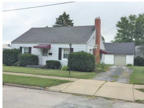
Before photo courtesy of 2018 applicant
