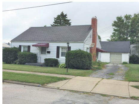
Before photo courtesy of 2018 applicant
