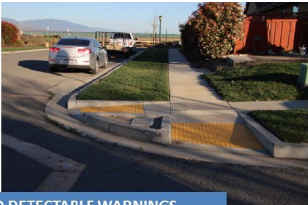
GOOD RAMP ORIENTATION AND DETECTABLE WARNINGS
