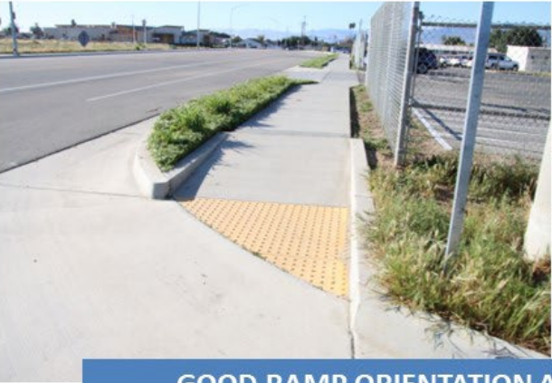
GOOD RAMP ORIENTATION AND DETECTABLE WARNINGS
