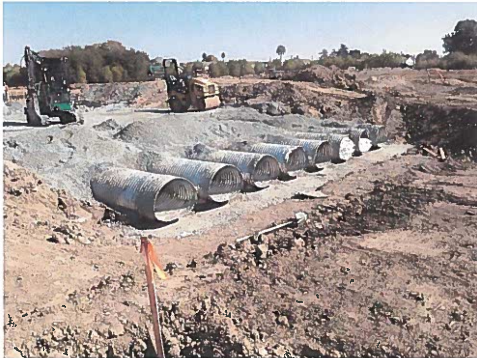
Floodway bypass culverts under construction
