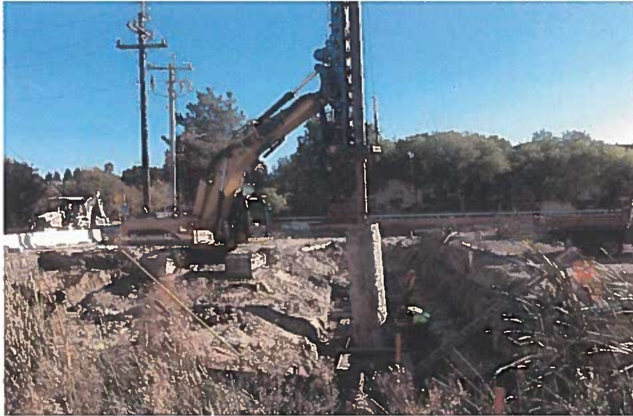
Drilling to pour bridge piles for the First Street Bridge at Rancho Vista
