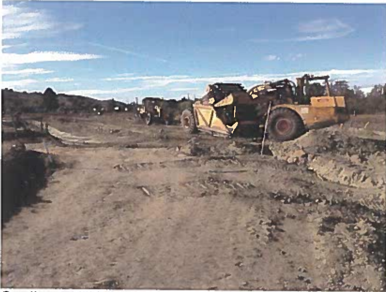
Grading activities continue in advance of curb, gutter and sidewalk
