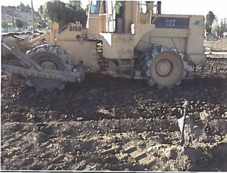
Compaction of the sub-grade in advance of paving.
