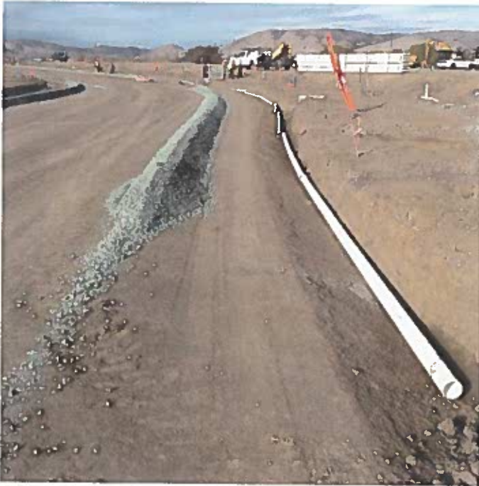
Drain piping under the curb and gutter.
