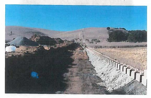
4. Finished aggregate base, and set finish grade at Rancho Way, Vista Way, Caetano Place, portion of Lavagnino Drive, and halfway of third Street which getting ready for the asphalt concrete on January 2, 2018
