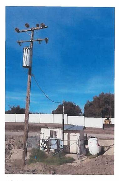
Well #2 abandonment waits for PG&E to remove the power drop and service pole from the well site. The Well would then be correctly abandoned and the site filled bring it to the new grade. The remaining interior street improvements could be installed.
