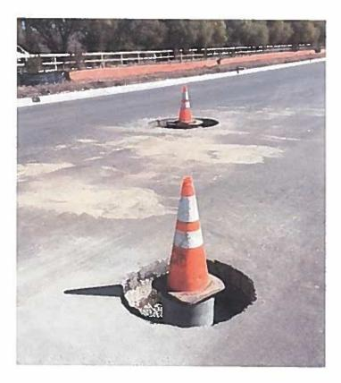
With the pavement being complete for the most part locating manholes and water valves are being raised to grade.
