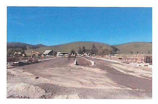
The construction of the main entrance to the housing tract continues toward completion with the placement of aggregate base on Levagnino Drive.
