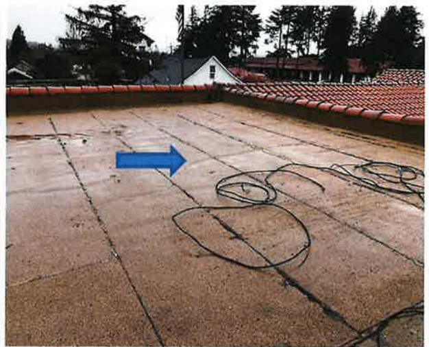
Picture # 5(continued) Roof has begun to blister.
