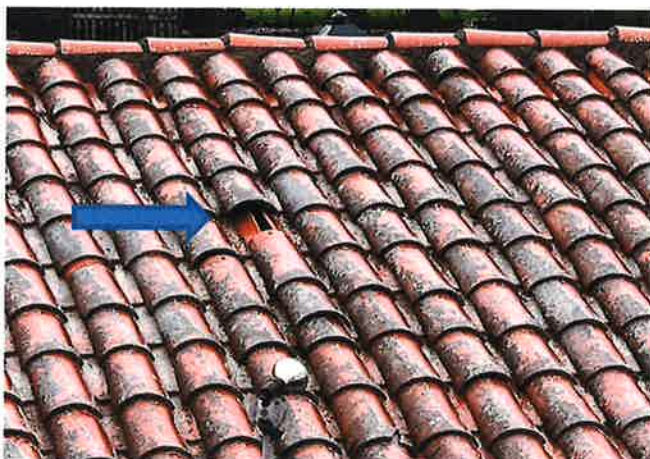
Picture #1 (continued) Missing tile, may cause leak if underlayment fails.
