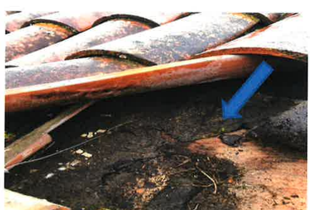
Picture #1 (continued) Deteriorating underlayment, plywood exposed continued.
