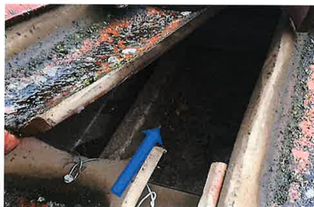
Picture # 4 Tile was overlayed on top of metal roof, no signs of water damage.
