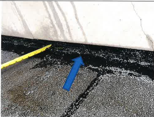
Picture # 5 Hot mop roofing has begun to crack.
