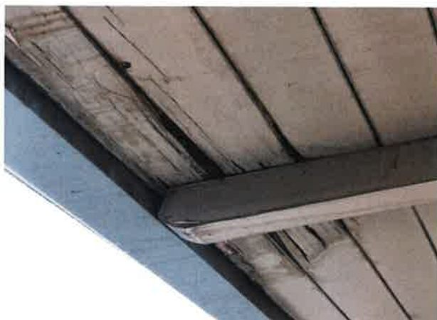
Picture #2 Most of the overhang beginning to rot due to underlayment failing.
