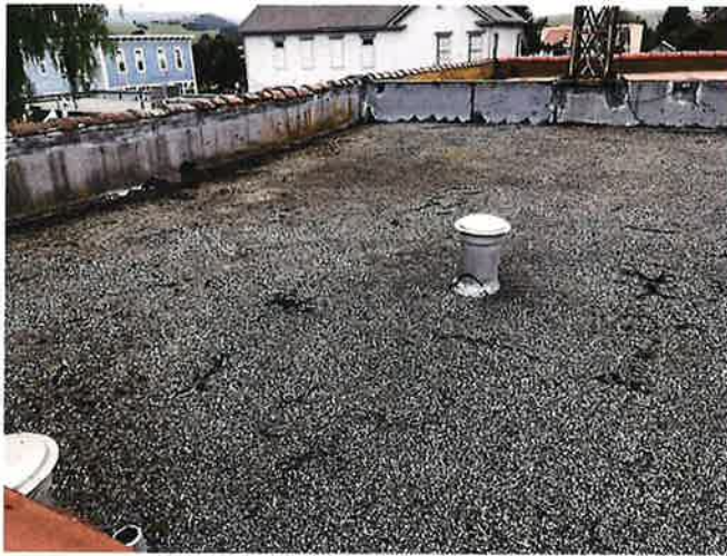
Picture # 5 Hot mop roofing has begun to crack.
