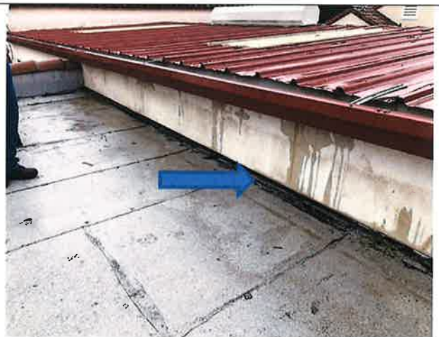
Picture # 5(continued) Roof has begun to blister.
