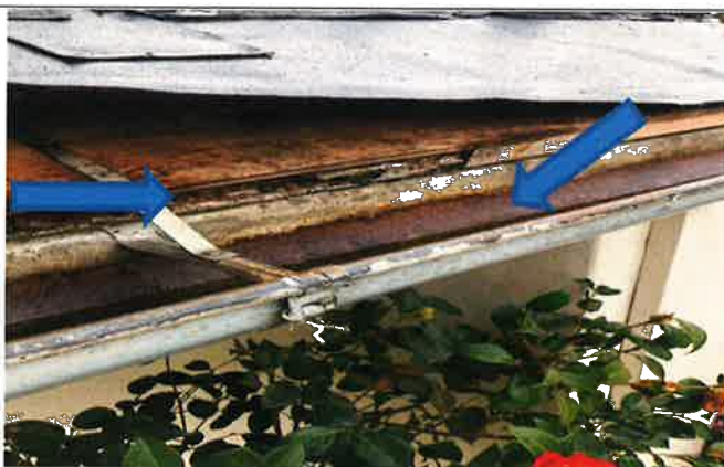
Picture # 3 Rotted plywood due to no edge metal, rusted gutters.
