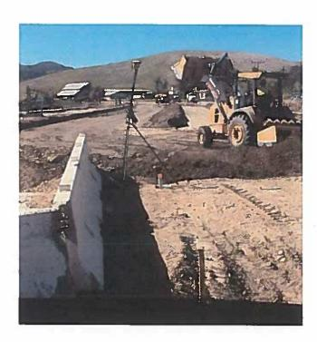
Backfill was placed around the bridge and compacted to required density. Contractor began installing concrete sidewalks and placing aggregate roadway base at 3rd St., Trailside Drive and Trailside Court. Stone walls were placed between lot number 7, 8 and 9.
