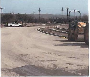
Grading and placement of base rock aggregate continued along Third Street extension a cross Lavagnino Drive to Rancho Way.
