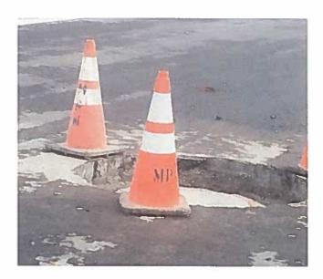
The water and sewer subcontractor began locating manholes and water valves, removing AC and aggregate base preparing to raise them to the new street grade.
