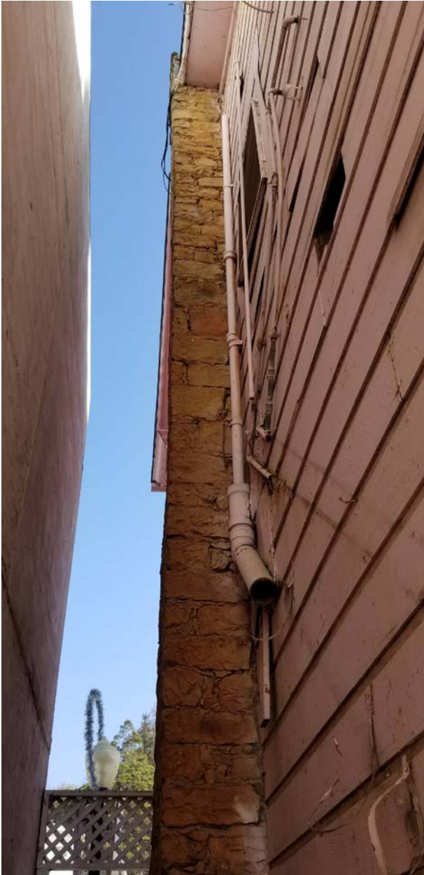
Unbraced unreinforced chimney at exterior.
