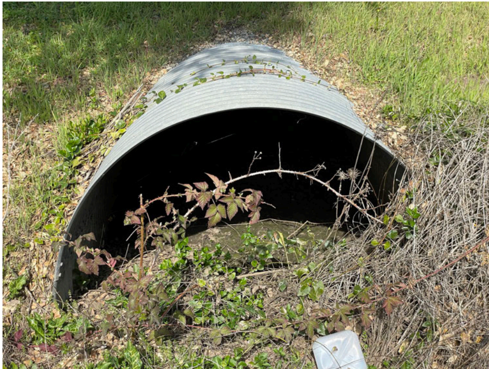
60-inch Culvert at Mission Vineyard Road (Upstream end)
