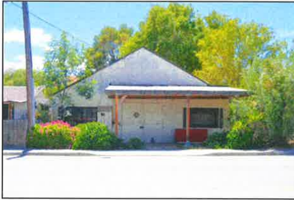
Figures 3 and 4. Left image shows the front (east) elevation. The stucco wall cladding was likely added in the 1950s. Right image details the north elevation, showing modern windows and replaced steel wall panels.
