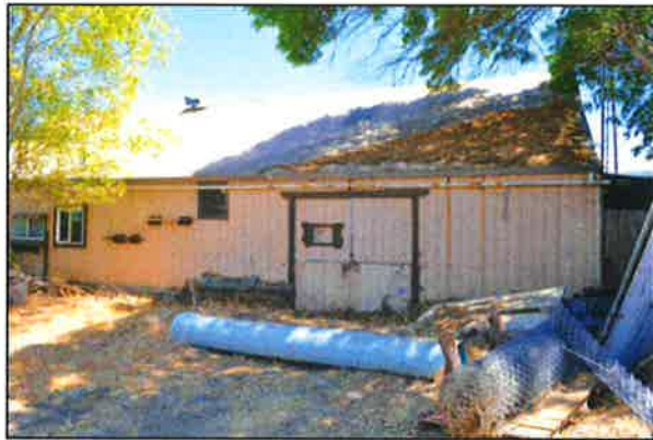
Figures 3 and 4. Left image shows the front (east) elevation. The stucco wall cladding was likely added in the 1950s. Right image details the north elevation, showing modern windows and replaced steel wall panels.
