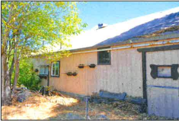
Figures 7 and 8. Left image details the north elevation, showing modern metal wall cladding and windows inserted into new openings. Right image details the rear (west) elevation, showing the detailing of the modern wall cladding system, window insertions and a poorly constructed rear addition.
