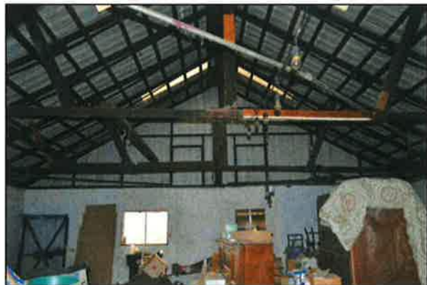
Figures 9 and 10. Left image details the interior looking toward the front (east) elevation wall. An arrow indicates the multi-pane window on the south side of the east elevation. Right image looks toward the west interior wall, showing rear trusses of a different configuration than the trusses located toward the front of the building. Note the interior plastering of the rear wall and the windows inserted into the wall.
