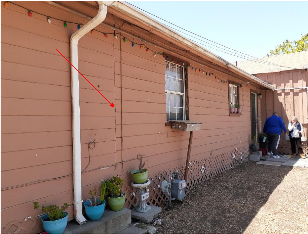
Figure 4: Arrow indicates change in siding
