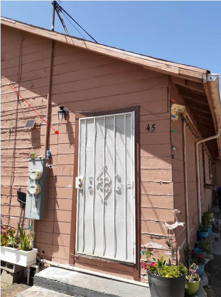
Figure 5: Arrow indicates change in siding
