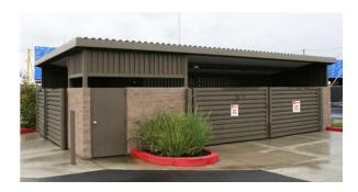
The *interior* dimensions of the enclosure are at least:  $(W \times H \times D)$ : 24' x 10' x 8' The width must accommodate three frontloading containers ("front loaders").
