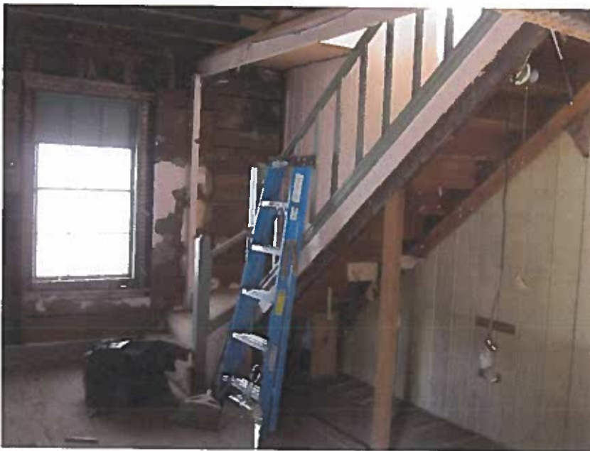
Figure 13: View of interior staircase to be removed within the main building, and window at the north elevation of the main building to be removed and blocked up
