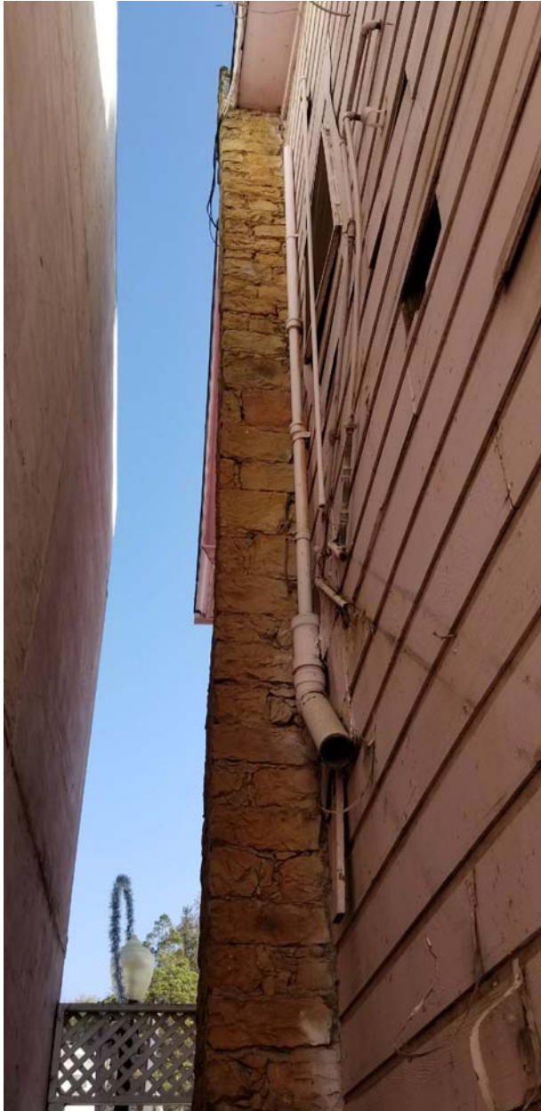
Unbraced unreinforced chimney at exterior.
