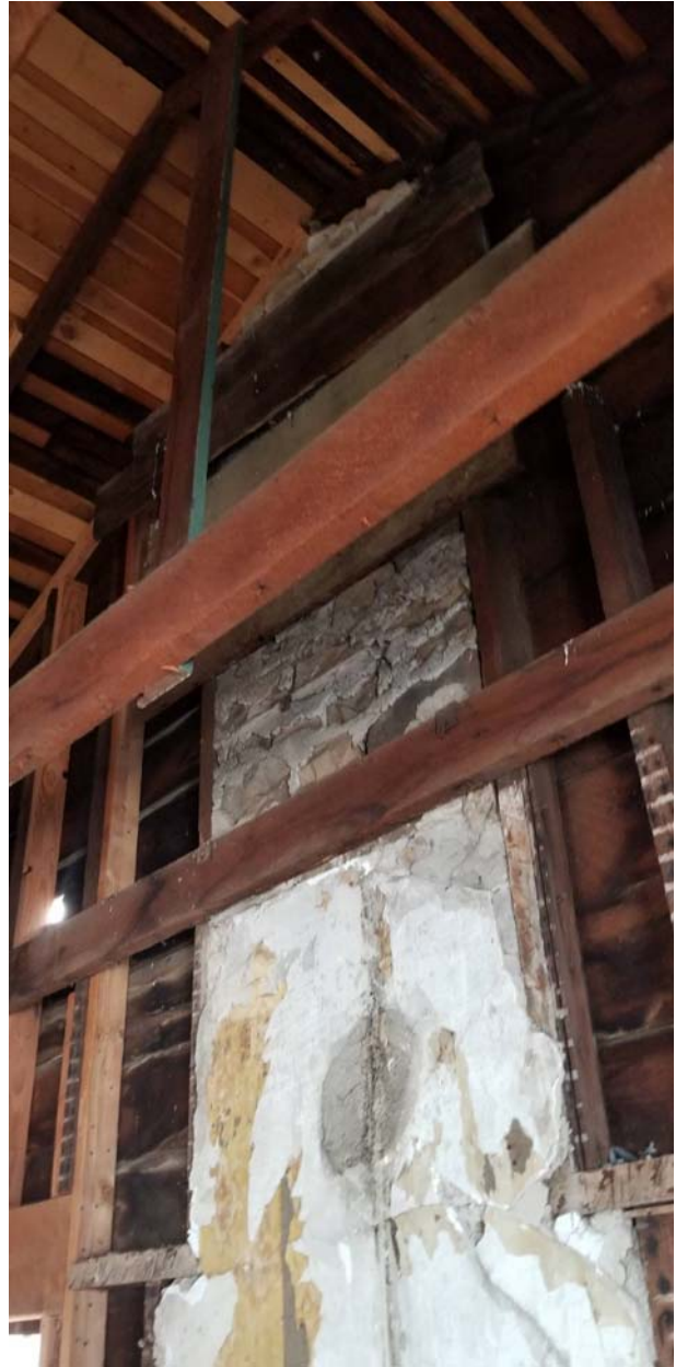
Unbraced unreinforced chimney at interior.
