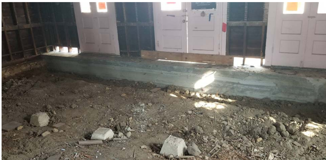
New foundation strengthening at front exterior wall. Note the demolished floor framing.
