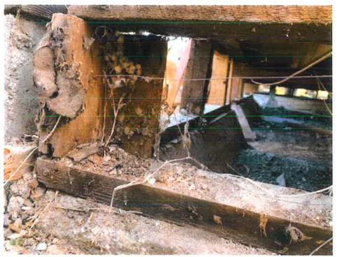
Figure 3: Evidence of foundation deterioration
