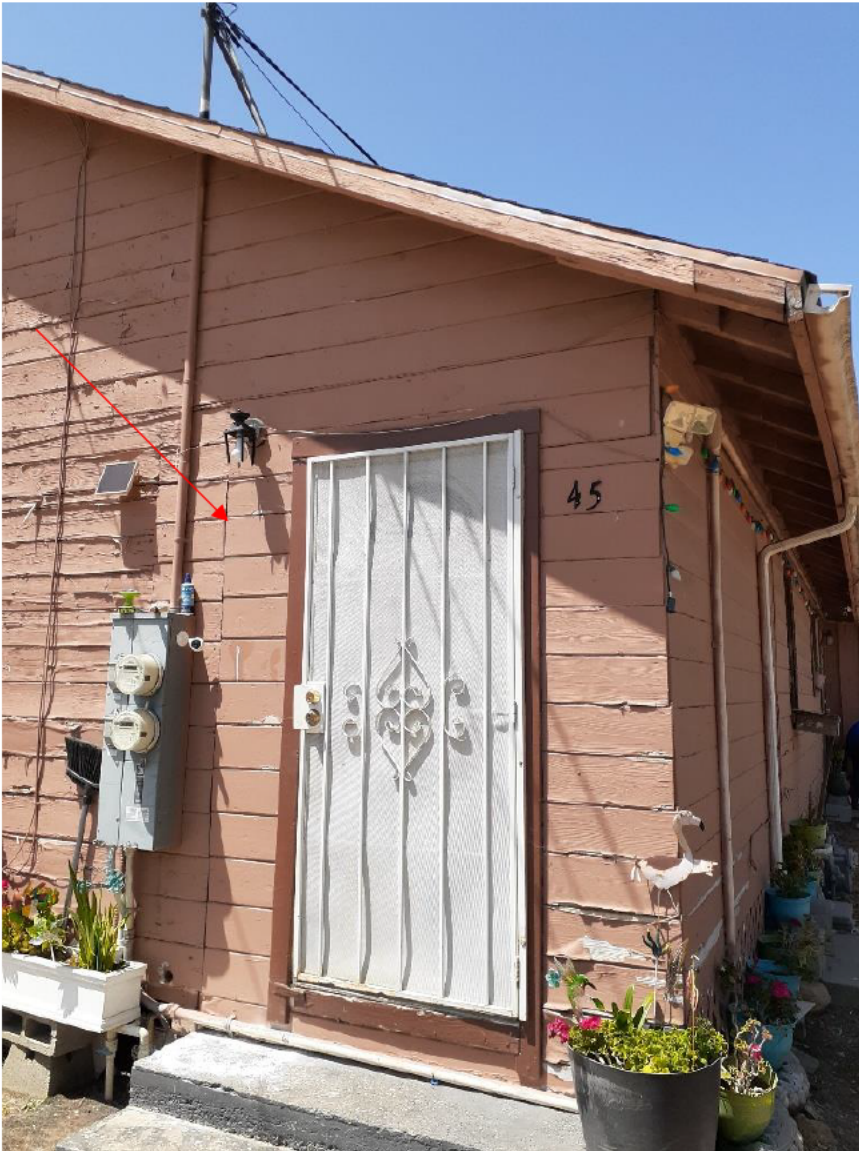
Figure 5: Arrow indicates change in siding
