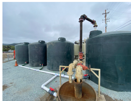
Well #6 Completed back wash tank Installation
