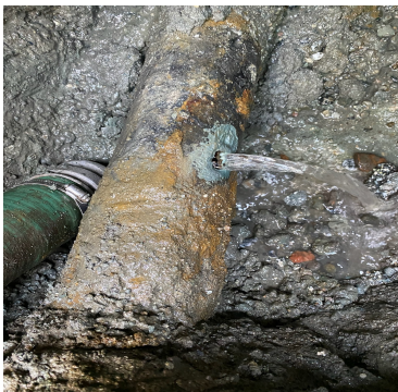
Alameda St/Pearce St water main leak
