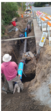
well 5 water main repair
