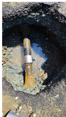
First /San Jose St Water main Repair
