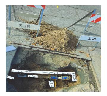
Water Main Repair North St / Second St . You can see the PG&E gas main right below the water main this is why we call USA North 811 to have other organizations utilities located so we can avoid hitting hazards with our equipment . We also found some previous repairs this section of pipe will be replaced during the valve replacement work.
