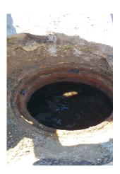
This manhole was found with our sewer camera and we went forward with excavating and installing a new frame and cover for future access for maintenance. This is located at the intersection of Merentis Circle / Monterey St
