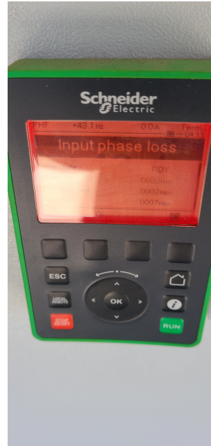
VFD error code well # 6
