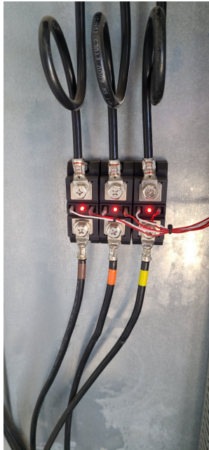
Failed safety relay Far right relay needed to be replaced
