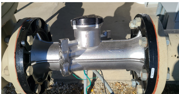
New Flow Meter well #5
