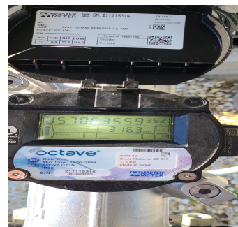
Flow meter register well #5
