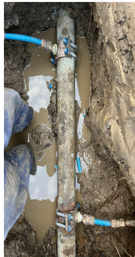
6th St water main repair
