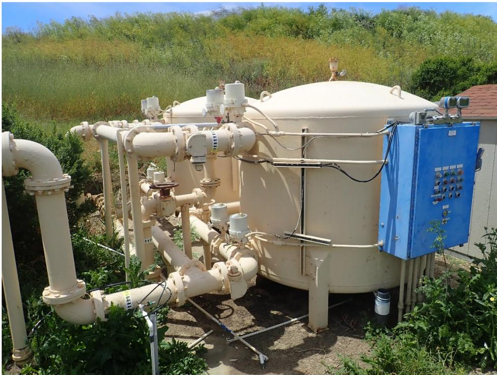
*Photo 14 : Pressurized filter system.*
