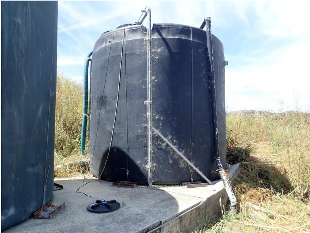
*Photo 7: The 10,000 gallon flow equalization tank located between Ponds on the far West side.*
