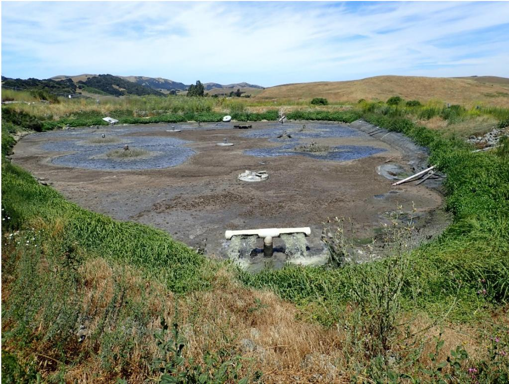
*Photo 5 : Pond 1, which acts as the sequencing batch reactor (SBR), from the East.*
