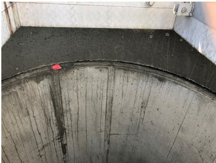
**Figure 5 – Possible Signs Of Infiltration Through The Concrete Joints**
