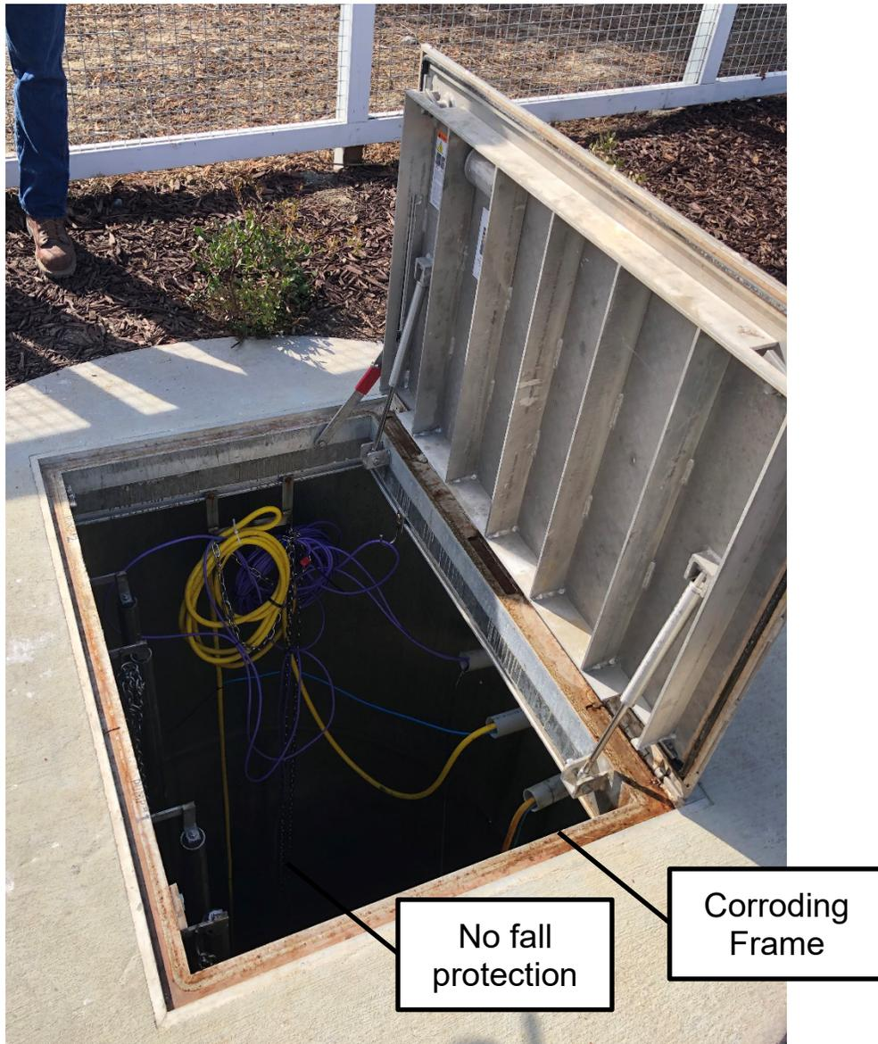
Figure 2 – RVSLs Wet Well Access Hatch
