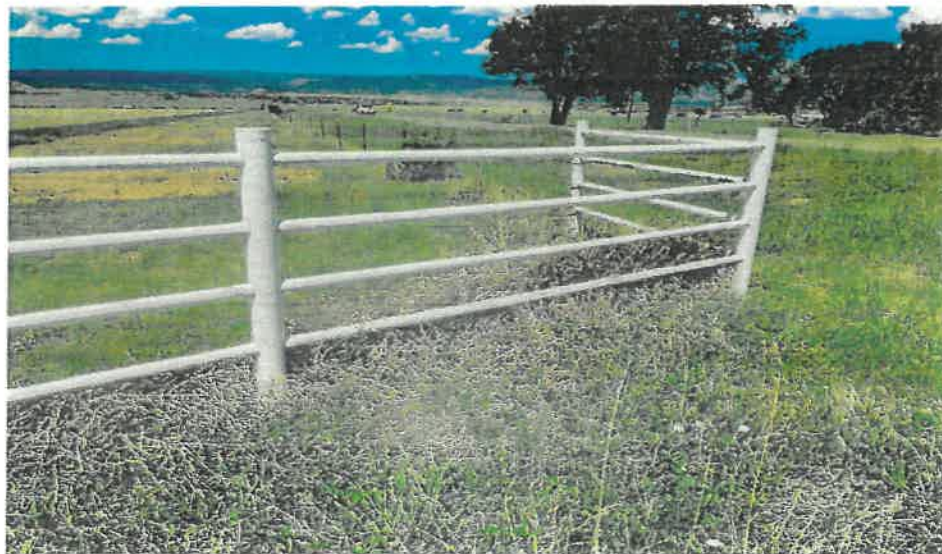
2" welded metal pipe entrance gate.
