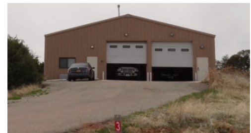
Village of Pecos Fire Station
