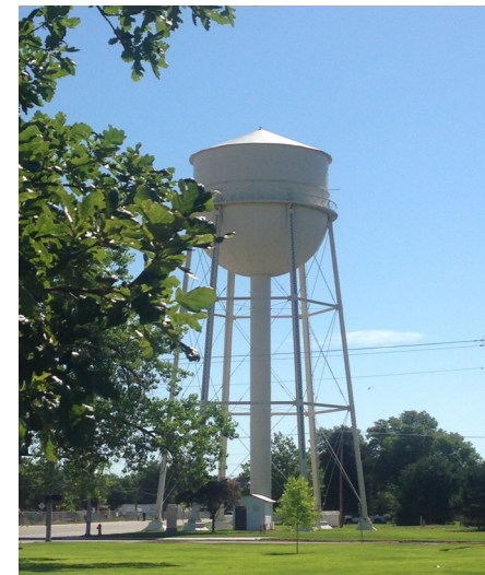
Water Tower - 27th Street & 2nd Avenue
