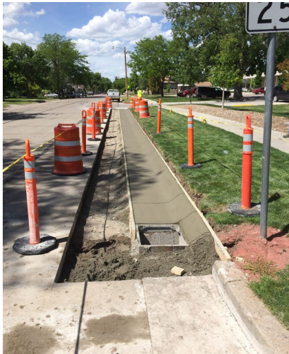
18th Street & 3rd Avenue
