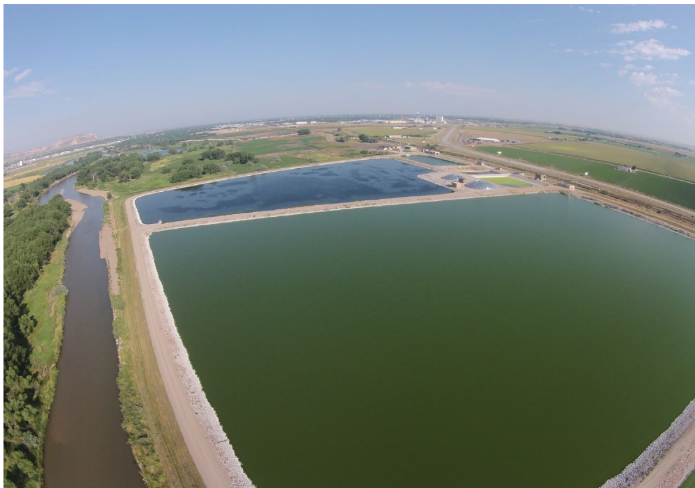
City of Scottsbluff, Wastewater Treatment Plant
