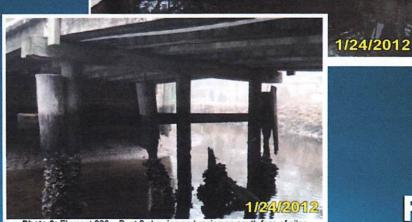
Photo 9: Element 206 - Bent 2 showing no bracing on south face of piles
