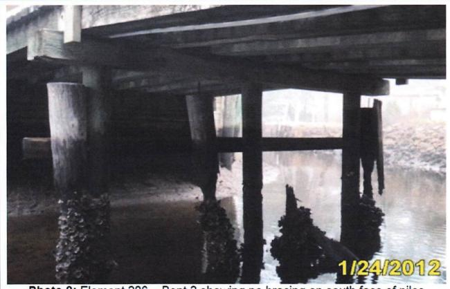
Photo 9: Element 206 - Bent 2 showing no bracing on south face of piles
