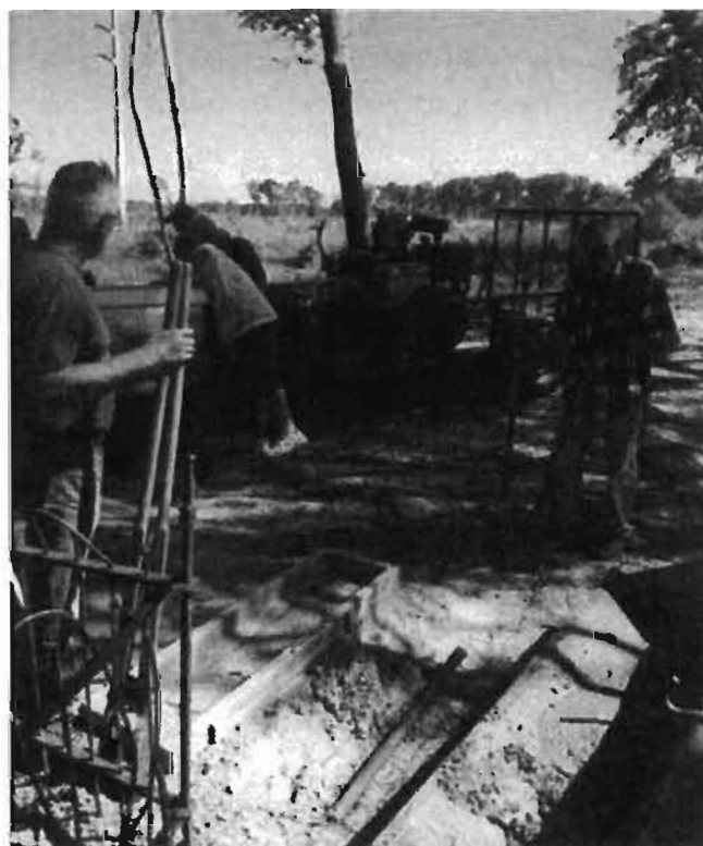
Construction of a Mold to Create the Cement Foundations for the Headstones
