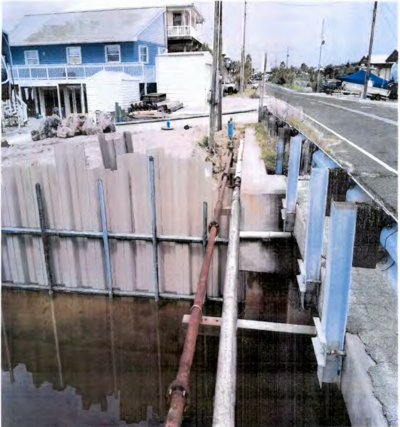
New seawall view from the canal
