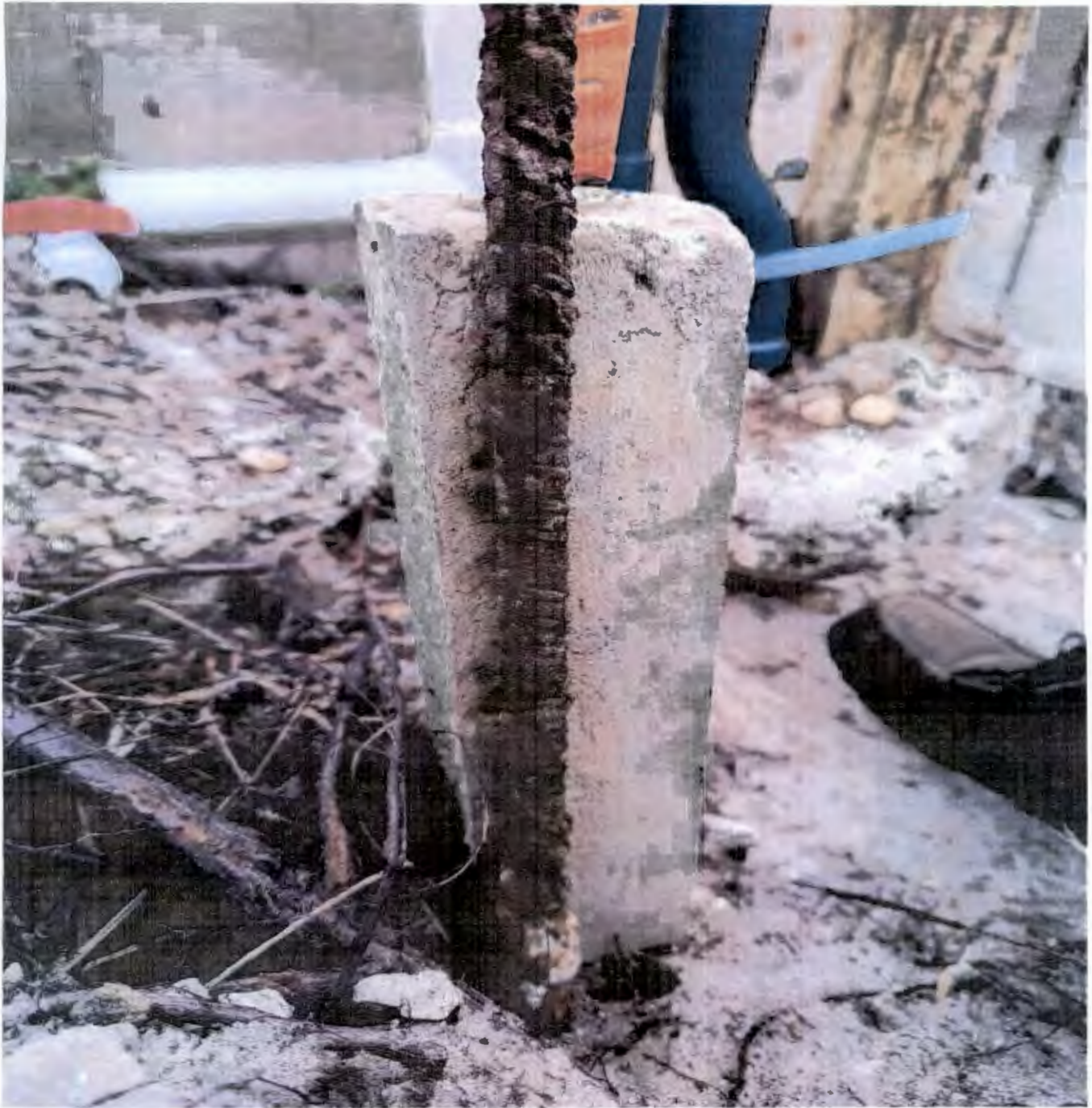
Rebar in place next to concrete monument
