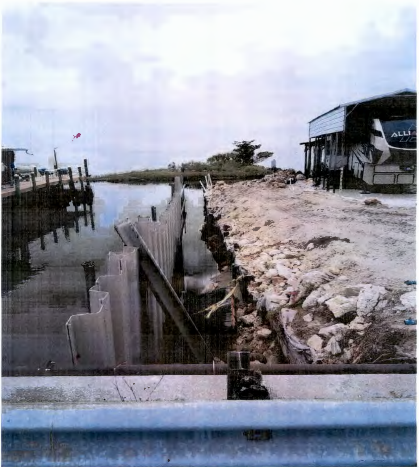
Existing seawall with new seawall installed approximately eight feet beyond the existing seawall.
