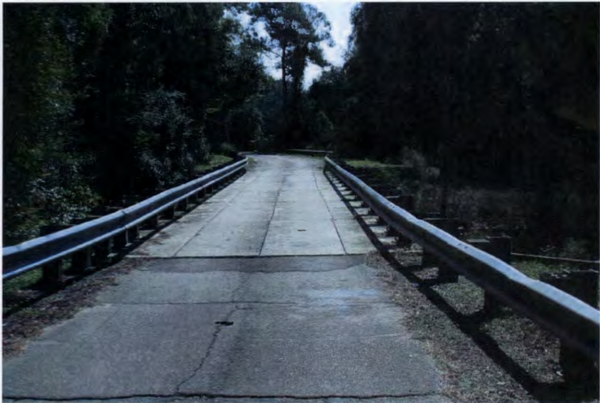
Overview of Bridge 384006 showing pre-cast deck panels and guardrail – note approach roadway shoulders are not carried across the bridge.
