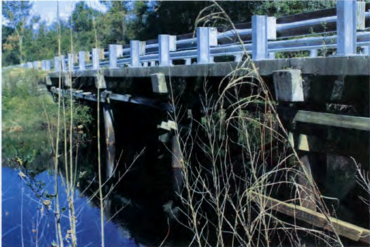
Side view of Bridge 384006 showing substructure with bracing members added. Note bracing creates a drift collection hazard.
