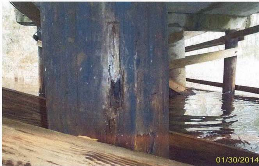
Photo 2 - Pile 4-2 hollow area and decay
