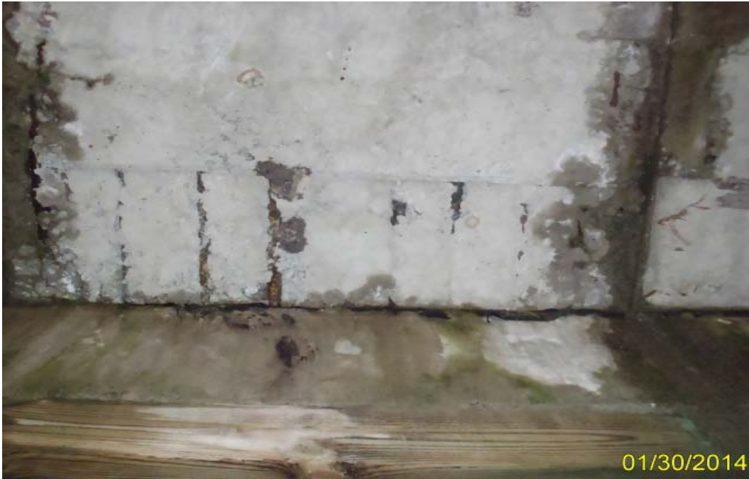
Photo 3: Element 38 – Honeycomb area with exposed rebar in deck underside of Slab Unit 3-2 at Bent 4
