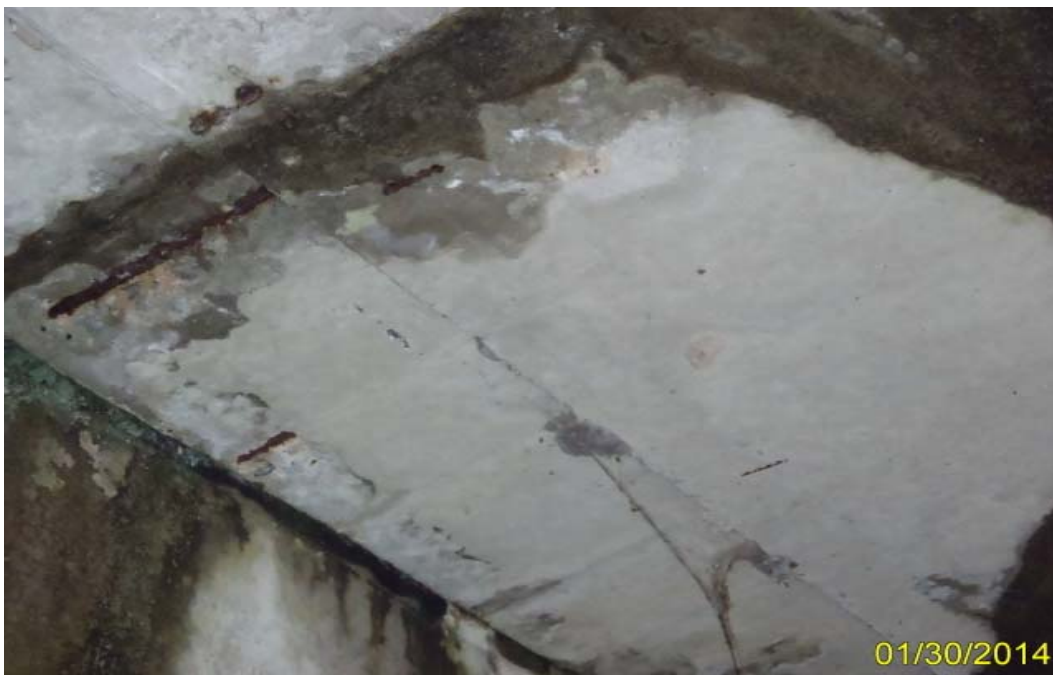
Photo 2: Element 38 – Exposed rebar due to lack of cover, Slab Unit 5-3 shown
