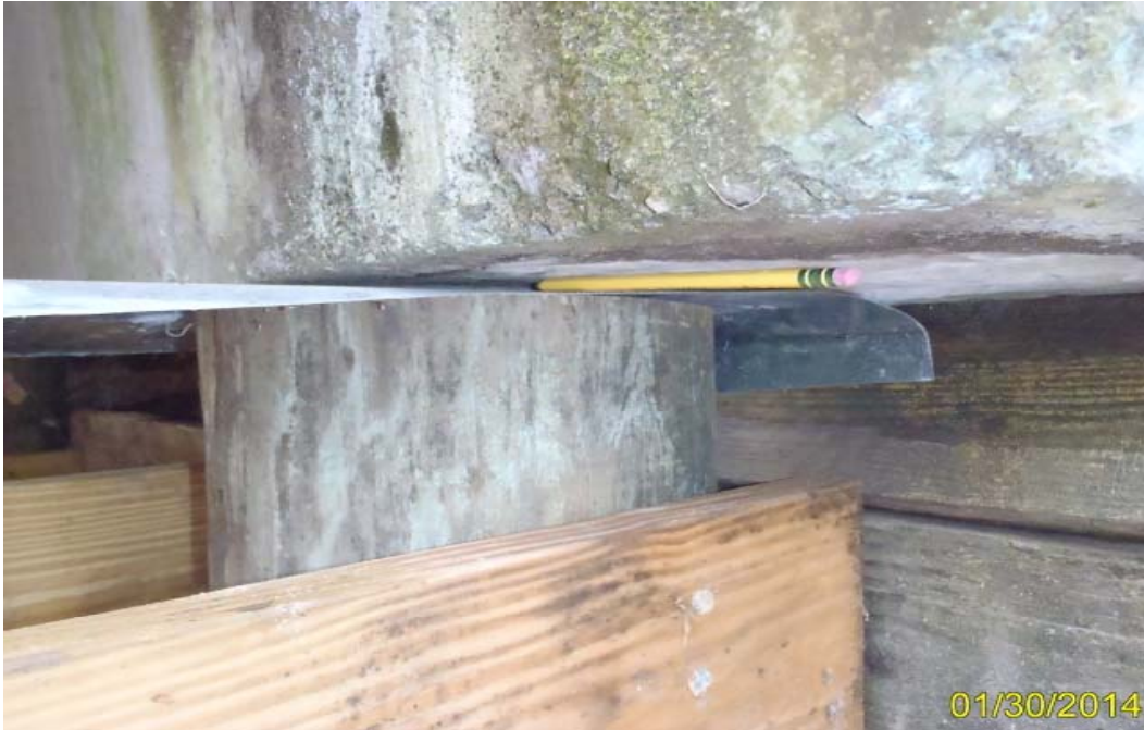
Photo 7: Element 215 – No bearing between Abutment 1 cap and Pile 1-1
