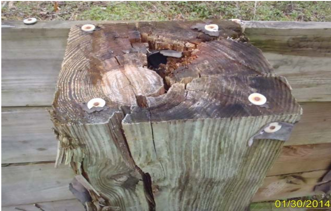
Photo 9: Element 476 – Deteriorated pile at the southeast wingwall
