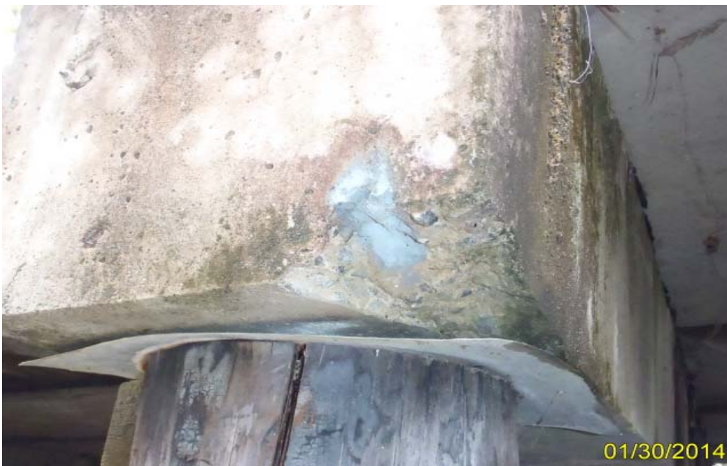
Photo 8: Element 234 – Spall with exposed rebar in the bottom southeast corner of Bent 2 cap.
