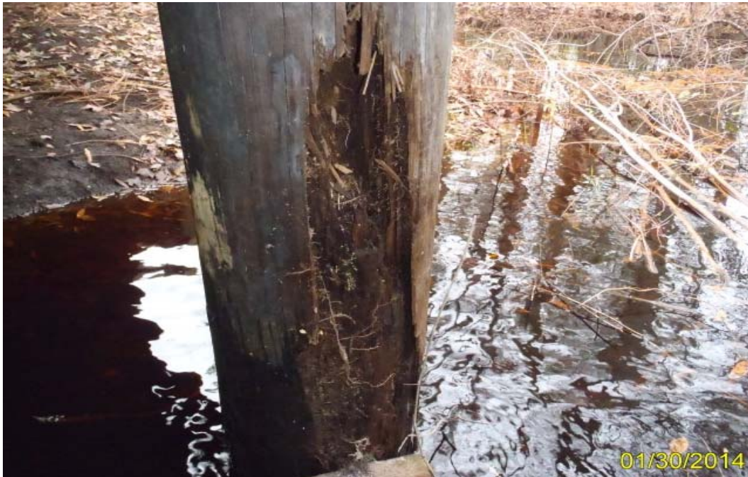
Photo 5: Element 206 – Pile 2-1 area of decay in the east quadrant
