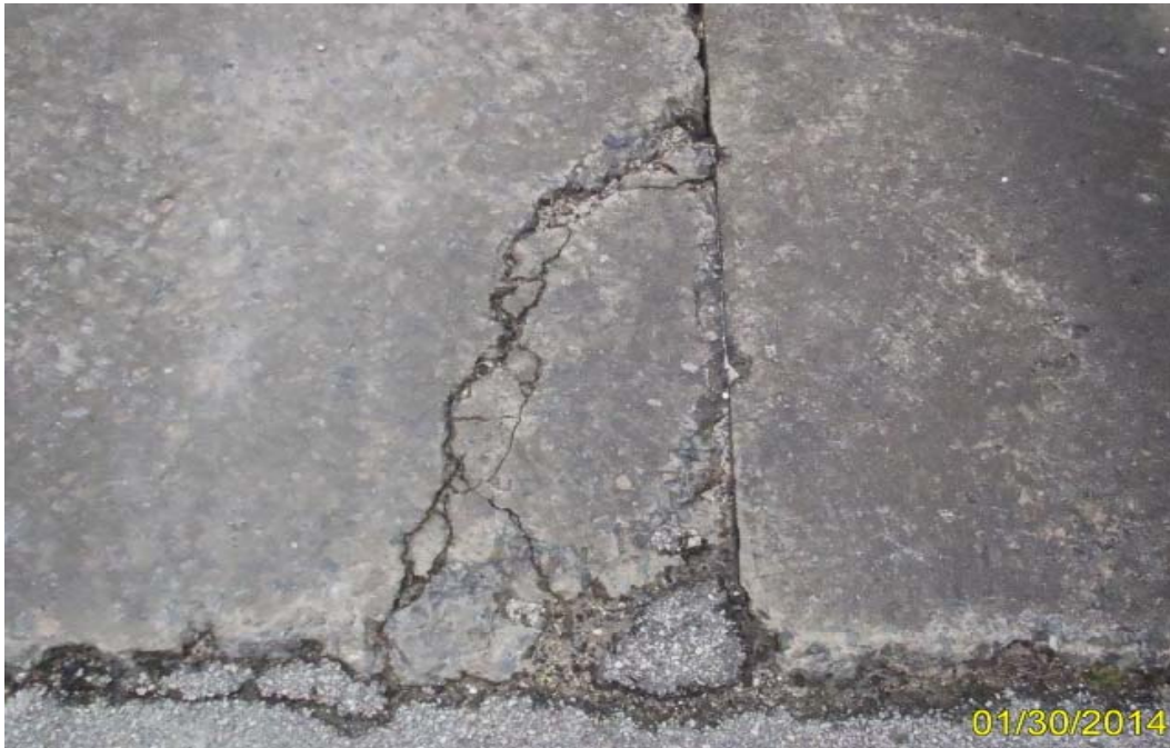
Photo 1: Element 38 – Delamination in deck top of Slab Unit 6-2 at the northeast corner
