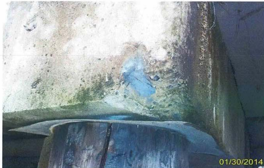
Photo 3 - Check in the south quadrant of Pile 2-4
