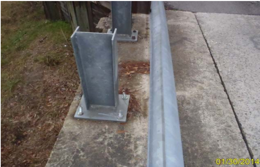
Photo 4: Element 334 – Missing cushion block for Post 1-2 Left
