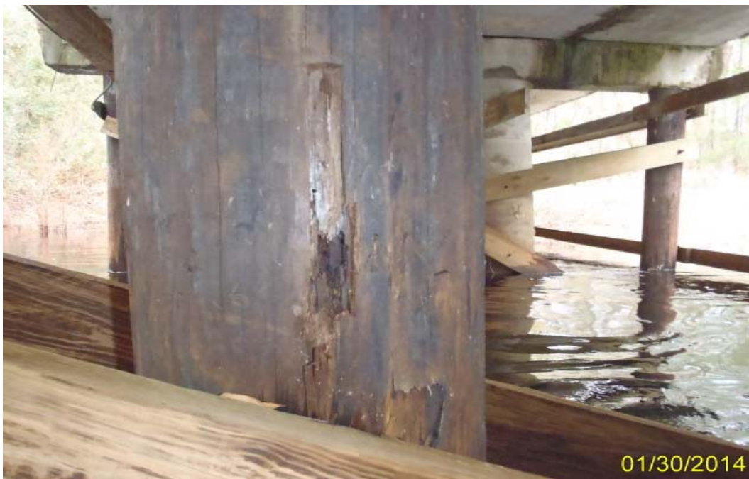
Photo 6: Element 206 – Pile 4-2 hollow area and decay
