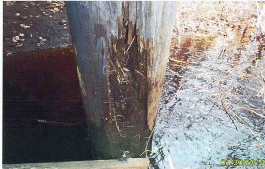
Photo 1 - Pile 2-1 hollow area and decay
